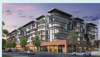
Project Name : Norwood Green – Stephenson Density: 43 Units Developer : Catcorp Projects / Buildtec Services / Aldi
